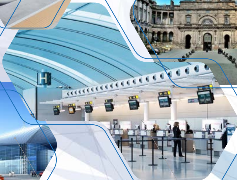
Airport in the capital of Mozambique
